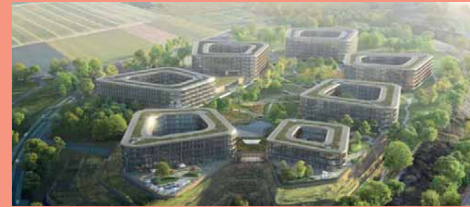
→ Office DE Schwarz Campus Bad Friedrichshall żagle sufitowe
